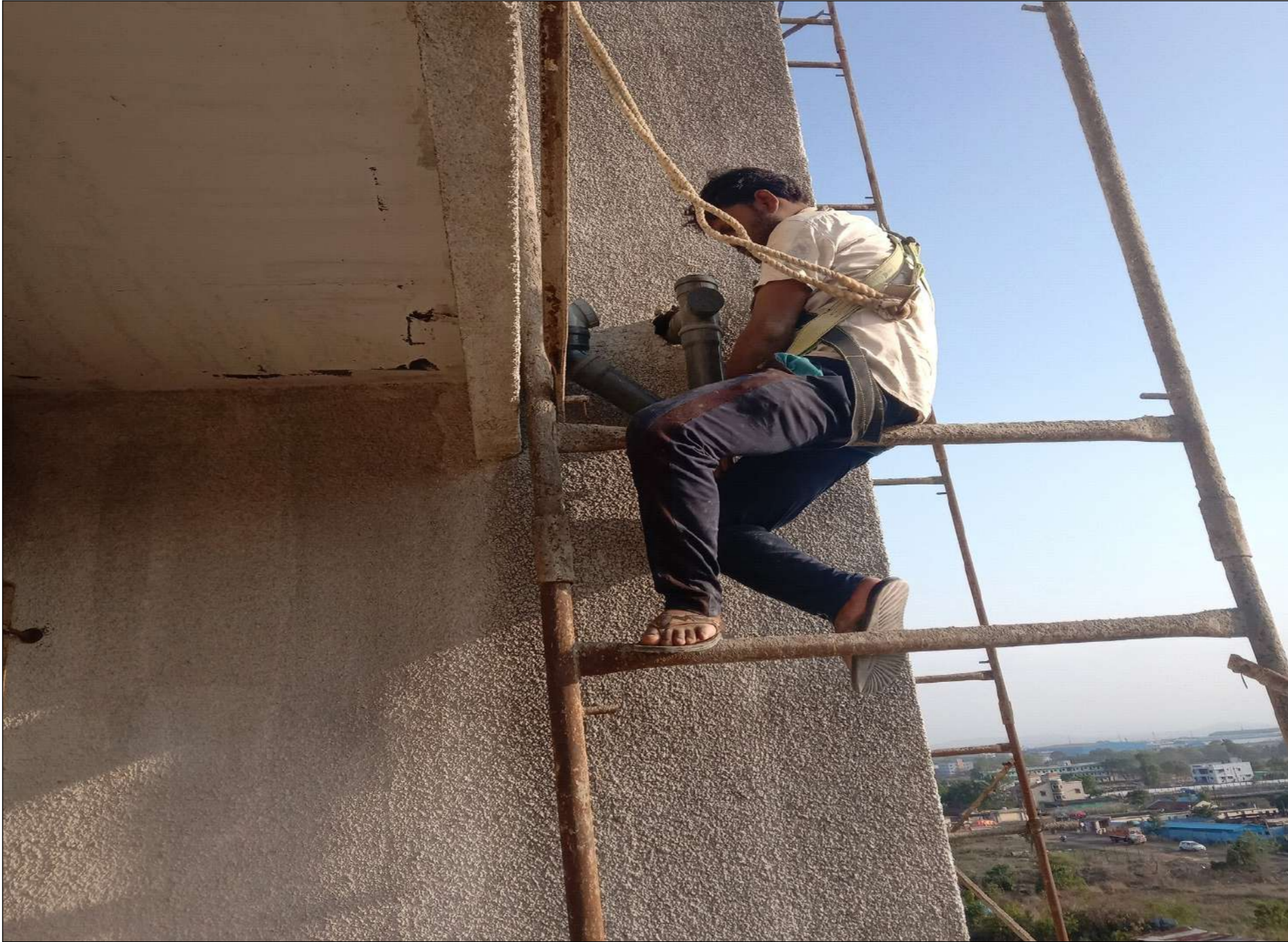
BUILDING C41: 7th FLOOR 2nd COAT PUTTY FINISHING WORK IN PROGRESS
