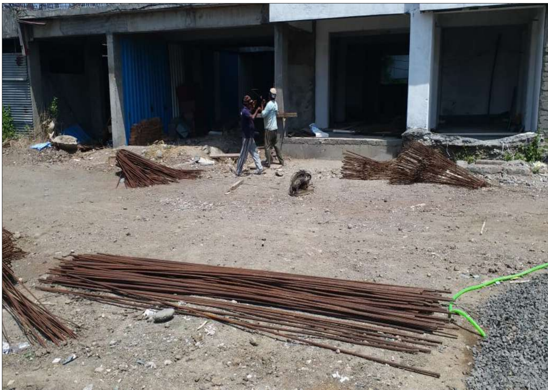
BUILDING C19, RET. WALL REINFORCEMENT CUTTING & BENDING WORK IN PROGRESS
