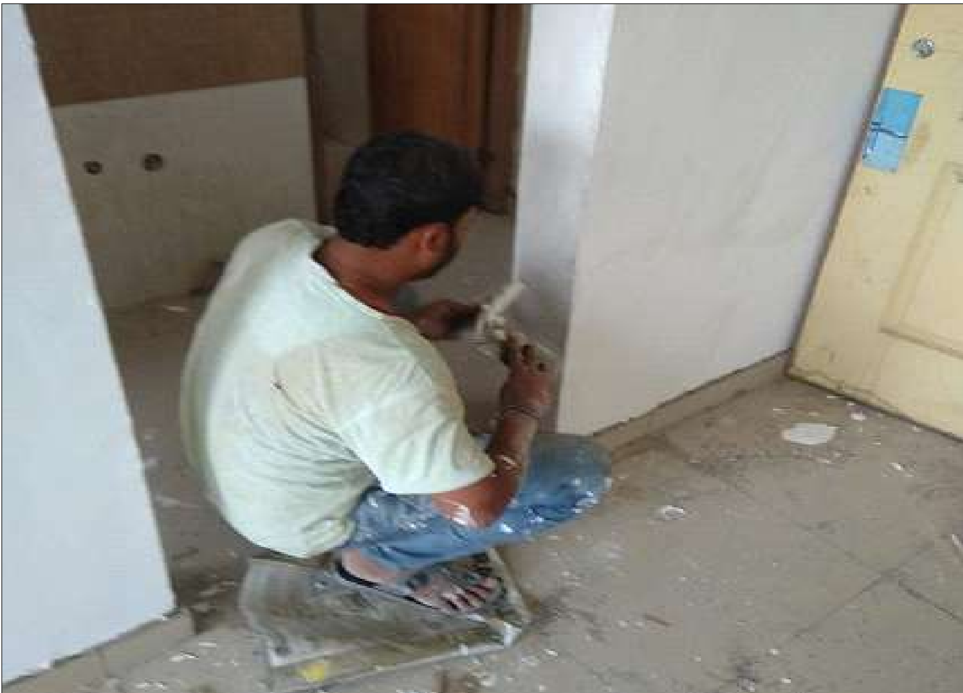
BUILDING C41: 7th FLOOR 2nd COAT PUTTY FINISHING WORK IN PROGRESS
