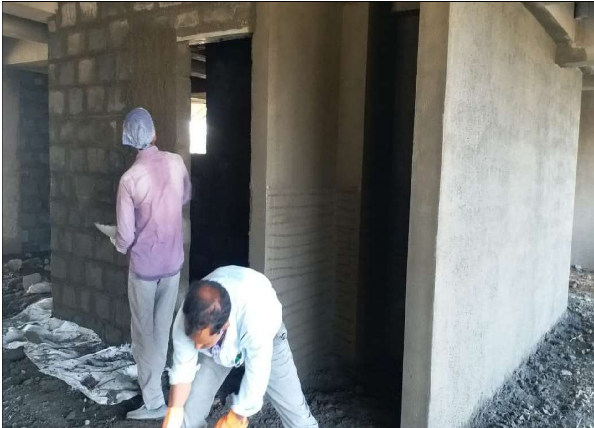
BUILDING C41, PARKING PLASTER WORK IN PROGRESS
