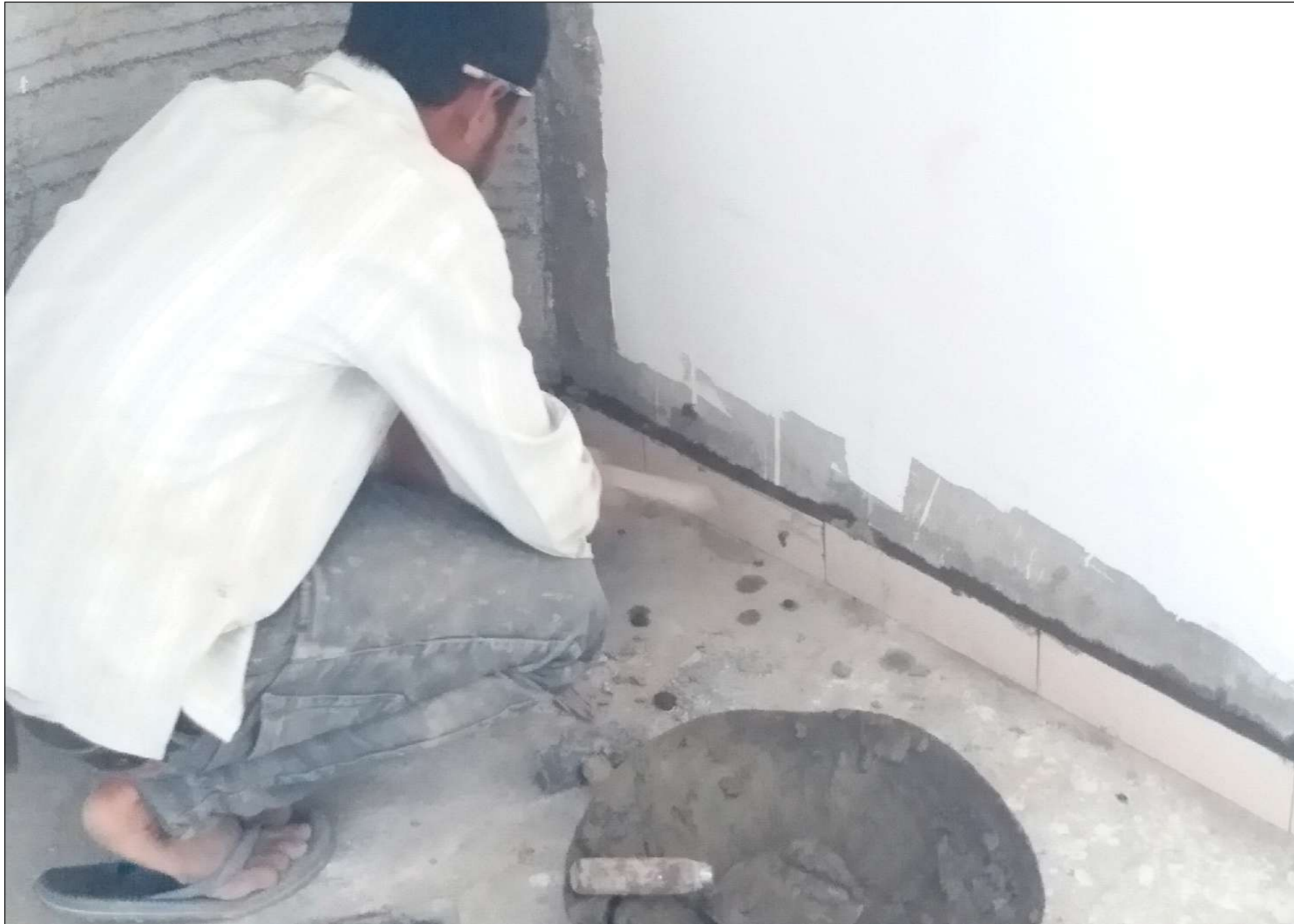
BUILDING C19, 11th FLOOR BALANCE KITCHEN OTA DADO FIXING WORK IN PROGRESS
