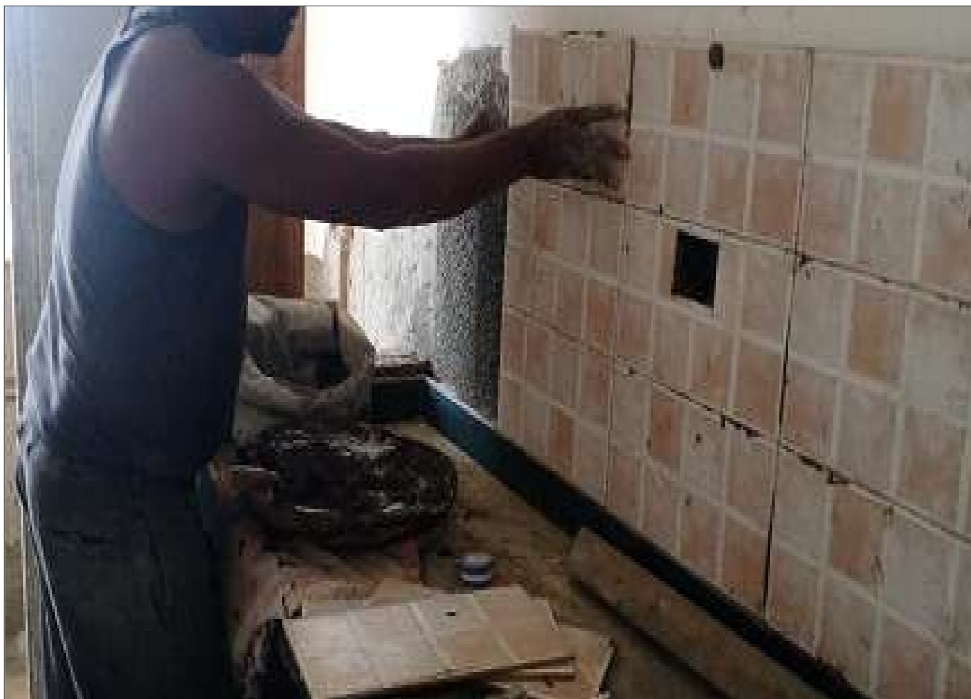
BUILDING C19, 11th FLOOR BALANCE KITCHEN OTA DADO FIXING WORK IN PROGRESS
